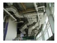
The severely compressed construction schedule required the mechanical and electrical design coordination effort be done while the structural steel was being erected, not a normal process for the construction industry. This deviation created many obstacles due to the ceiling space limitations. Since the building structure could not be altered to create more ceiling space the mechanical/electrical design changed daily, requiring the ductwork to also change daily.
