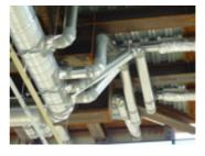
Finger lines go to the slot diffuser that feeds the gallery rooms in the new wing.
