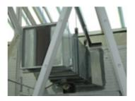
Sixteen smoke evacuation systems were installed in the attic of the 1916 building taking care not to damage the original skylights overhead.
