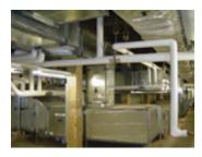
The ductwork was strategically placed between the original columns in the 1916 building's mechanical equipment room.
