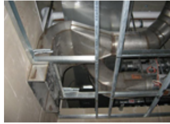
Fully welded round and rectangular stainless steel distribution systems.
