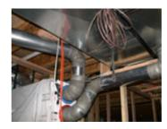
Note that both the supply and return air duct are ducted. All the duct joints were sealed with mastic.
